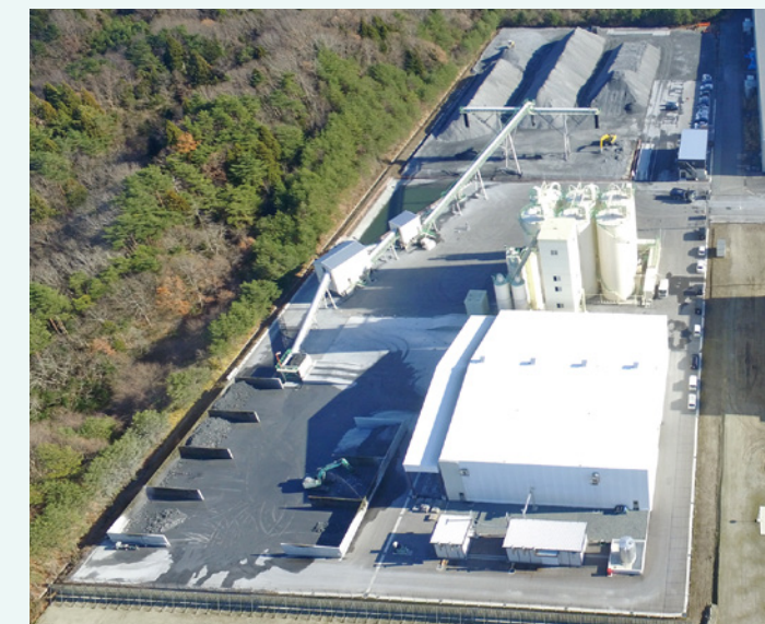
Entire view of Fukushima EcoCrete Plant
