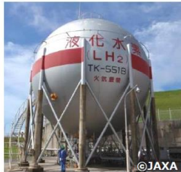
LH2 Storage Tank at Tanegashima Space Center
