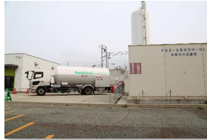
Filling a storage tank with hydrogen
