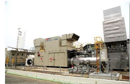
Hydrogen CGS demonstration plant
