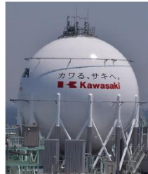
Japan's biggest LH2 Tank at Kobe LH2 Terminal
