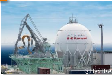
Storage Tank at Hy touch Kobe: 2,500m 3
