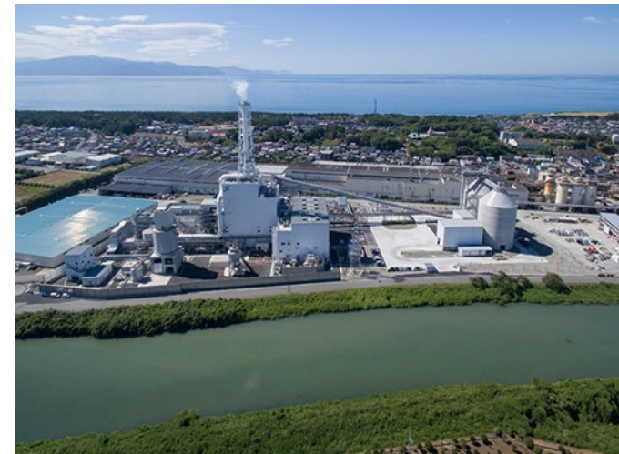
Suzukawa Energy Center Power Station
