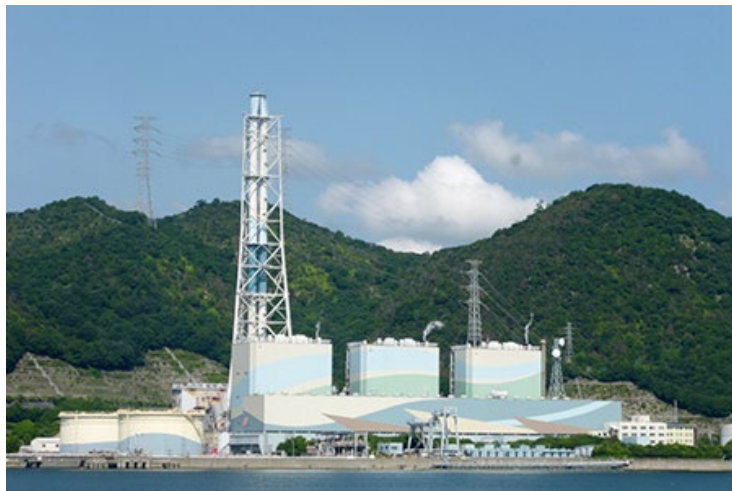
KEPCO Aioi power station
