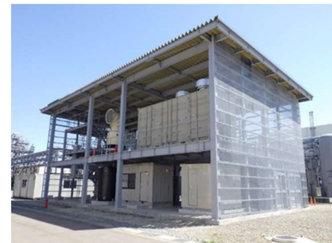
Methanation test facility
