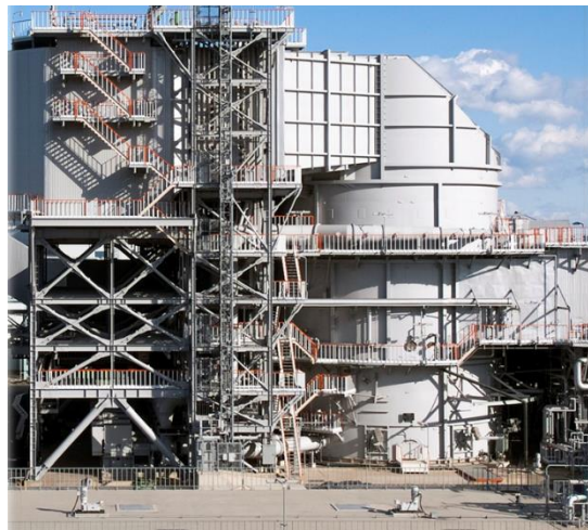
Figure 26. Limestone Gypsum Method FGD (Source: Mitsubishi Power)
