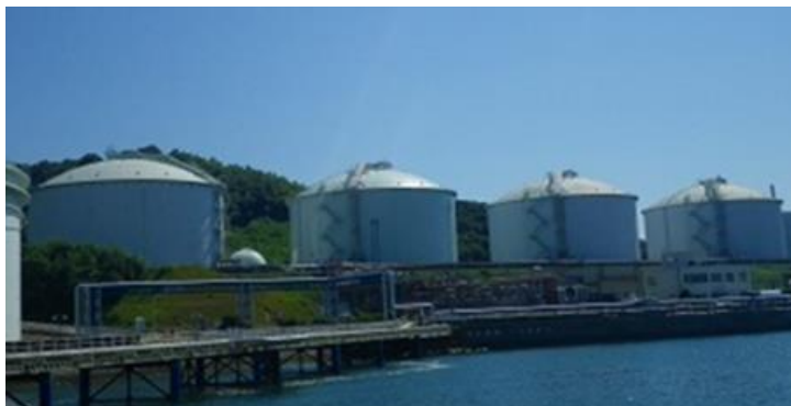
LPG Tanks (Refrigerated Storage Tanks)
