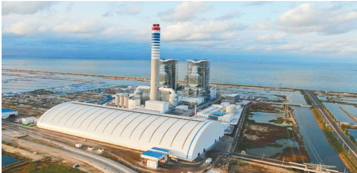
Datang Dongying Power Generation Co., Ltd Million-kilowatt ultra-supercritical coal-fired power unit
