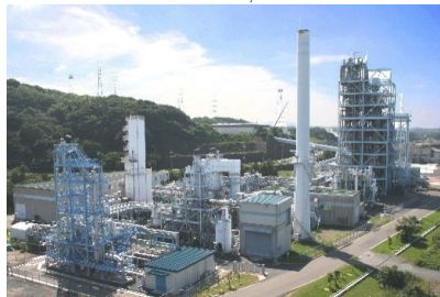
Demonstration test of oxygen-blown coal gasification and CO 2 separation and capture
