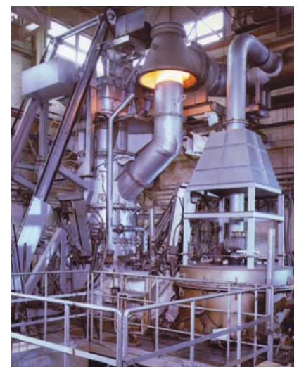
Fig. 2 Pilot plant (6t/hr)
