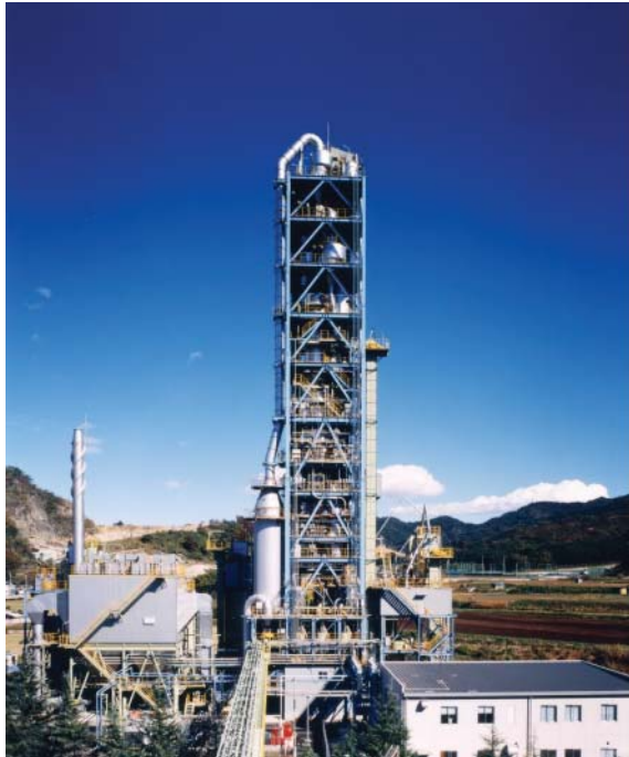
Photo 2 Overview of 200 t/day plant
