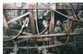
Gas drainage hole
