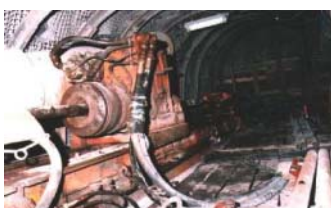
Gas drainage boring
