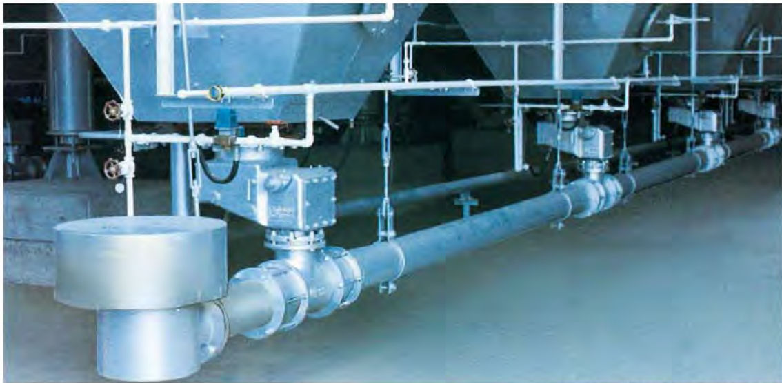
Adjustable Air Intake and Fly Ash Intake
