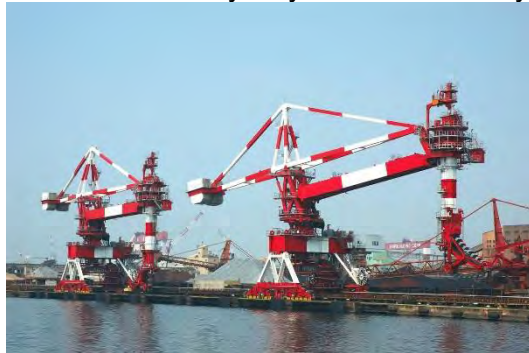
Figure 78. Bucket Elevator Continuous Ship Unloader (CSU) 1
