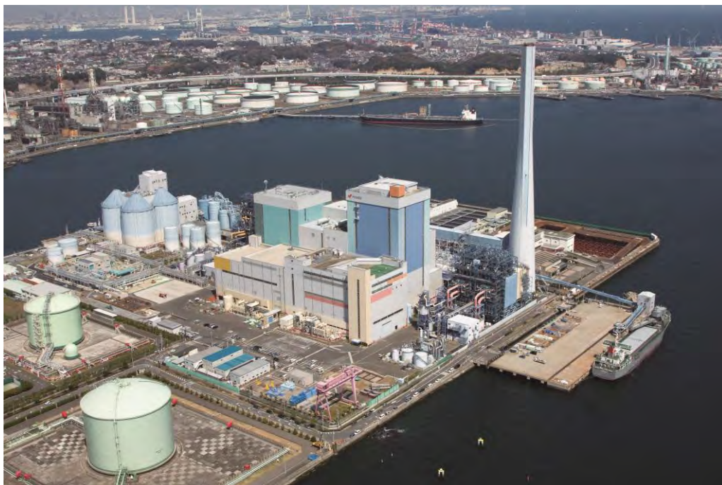
Figure 44. Up-to-date USC, Isogo No. 1, and No. 2 Units
