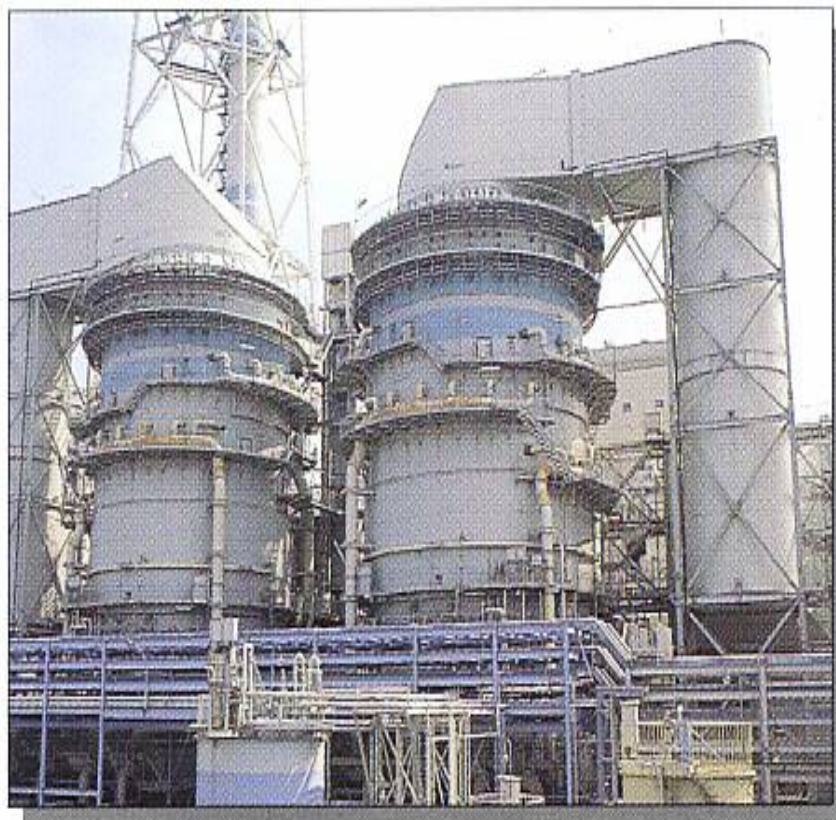
Matsuura Thermal Power Station
